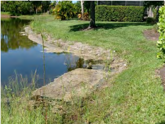
Sod replaced on lake bank
