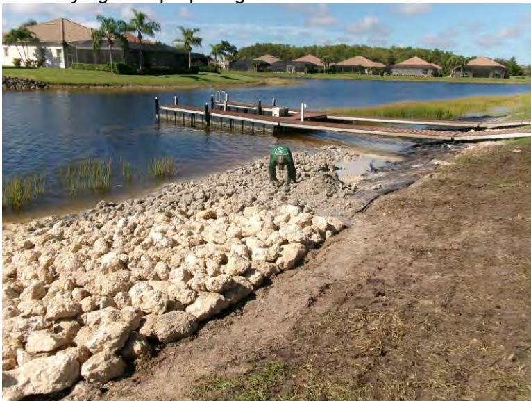
Crew laying the riprap on geotextile
