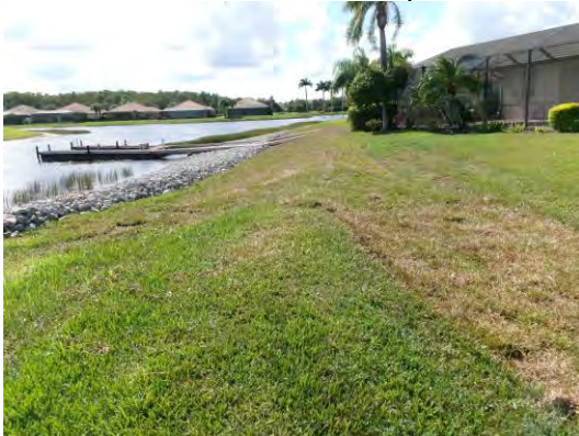
Sod laid down on skid steer path
